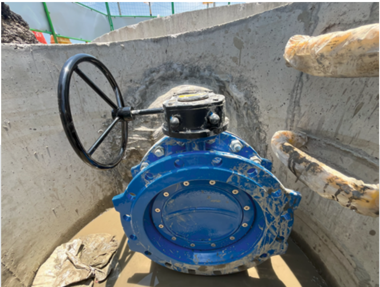
Butterfly valve installed
